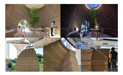
*Figure 3.* The result of research in 3D printing and architecture of the Italian company GAIA (2020)
